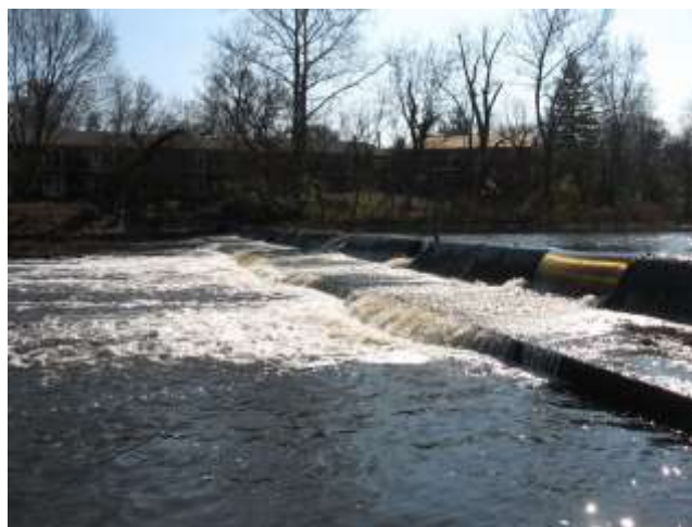
Former Low Level Dam at Batavia
